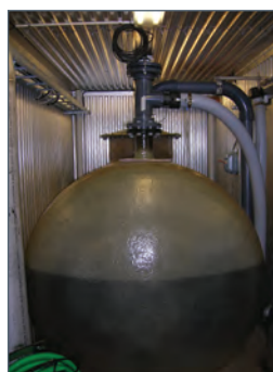
CHEMICAL TANK WITH STANDPIPE 1.9m (6ft)
