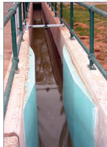
RECTANGULAR FLUME FLOW
