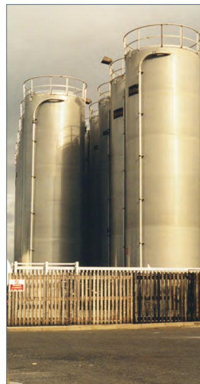
PLASTIC PELLET SILOS 18m (60ft)
